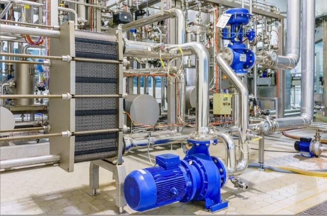
The great advantage of our plate heat exchanger lies in its easy maintenance and flexibility to adapt to any production requirements. Due to different board ripples, various possible nominal connection widths and different heat lengths, we always provide correct and economic solutions for your application.
