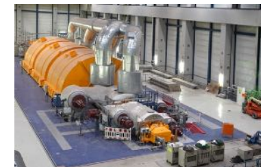
A turbine generator
