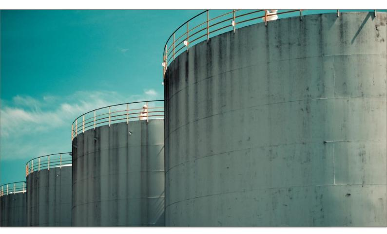
Generally speaking, the receiving terminal should have at least 2 tanks of equal volume. For example, this scheme accepts that the scale of the first phase of the terminal is 2.0 Mt/d, and the LNG carrier used is 135,000 m<sup>3</sup>. If the number of consecutive non-operational days is 5d and the unloading time is 12h, the 135,000 m<sup>3</sup> LNG carrier should be selected.
