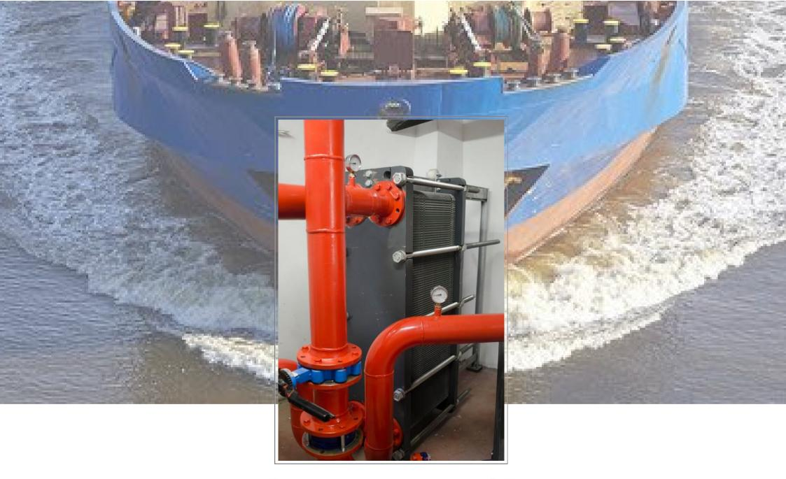
The heat transfer area of plate heat exchanger (PHE) achieved by the same volume is 5-10 times that of the shell and tube heat exchanger, and it is easy to dismantle and clean. The compact design structure makes it perfect for the marine vessels.
