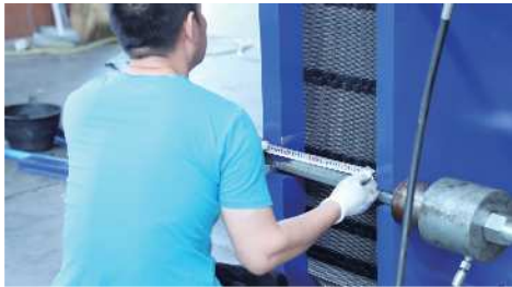
Inspecting and adjusting the tightening dimensions of a Plate Heat Exchanger
