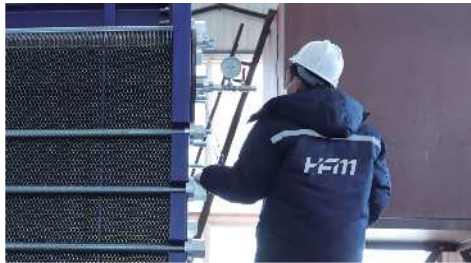
Pressure testing procedure of a plate heat exchanger
